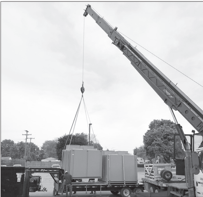
New HVAC Installation at Warren Woods Middle School
