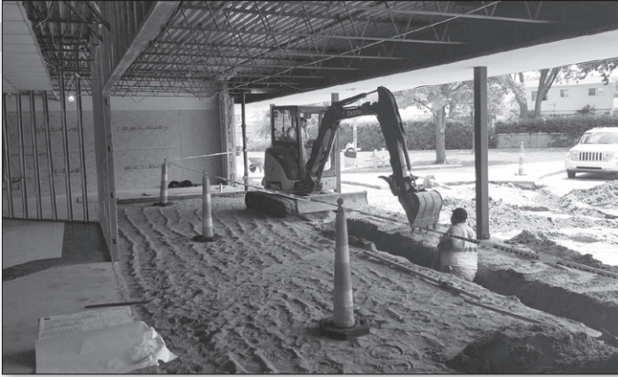
Pinewood Elementary Secure Entry
