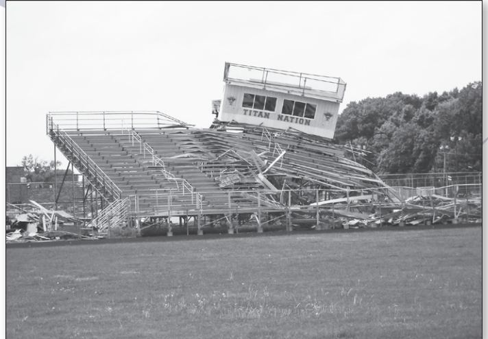
Demolition of bleachers at Warren Woods Tower
